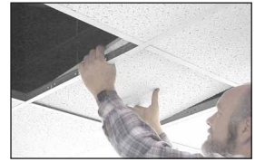
Remove two ceiling tiles.
