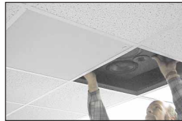
Slide the loudspeaker onto the grille.
