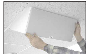
Snap on the grille and replace the second tile.
