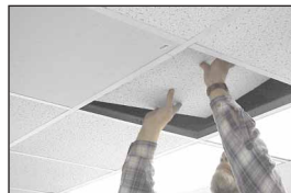
Replace the second tile.
