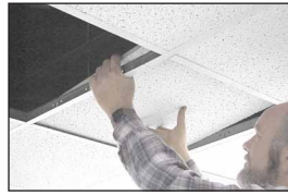
Remove two ceiling tiles.
