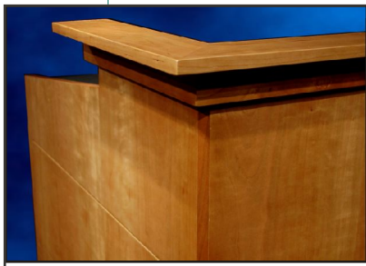
A deep reveal creates smooth shadow lines
