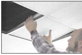
Remove two ceiling tiles.
