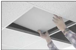
Place the grille into the first opening.
