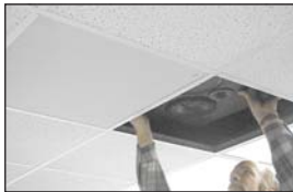
Slide the loudspeaker onto the grille.
