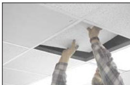
Replace the second tile.
