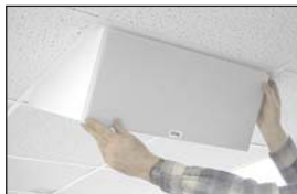
Snap on the grille and replace the second tile.
