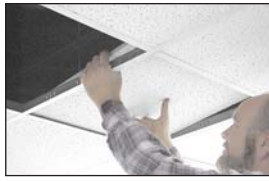
Remove two ceiling tiles.
