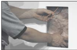
Fish the wire and add fiberglass.
