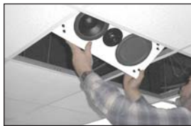
Slide the loudspeaker through the opening. Make sure that it fits flush.
