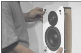
Slip the loudspeaker into the opening.
