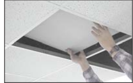
Place the grille into the first opening.
