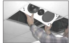
Slide the loudspeaker through the opening. Make sure that it fits flush.
