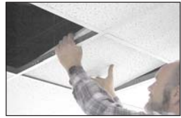
Remove two ceiling tiles.
