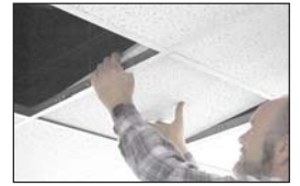
Remove two ceiling tiles.
