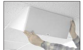
Snap on the grille and replace the second tile.
