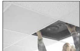
Slide the loudspeaker onto the grille.
