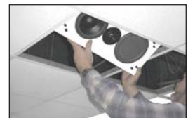
Slide the loudspeaker through the opening. Make sure that it fits flush.
