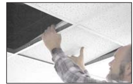
Remove two ceiling tiles.
